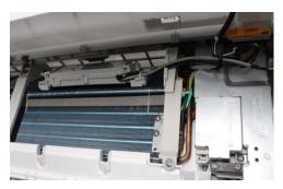
Fig. 33 — Use ties to keep wiring aligned
