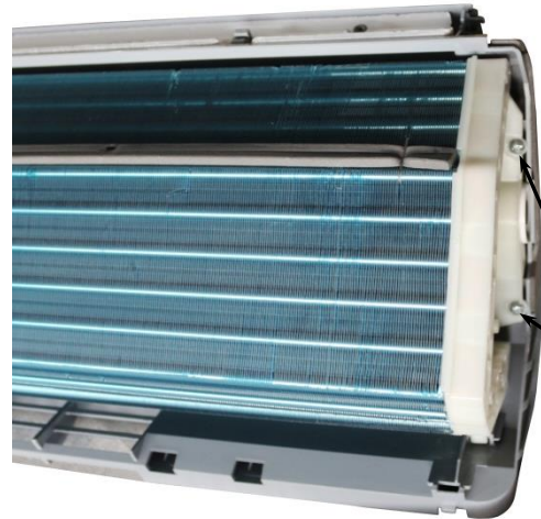
Two screws at the base bearing side
