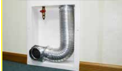
② Clean finish leaving room for duct
