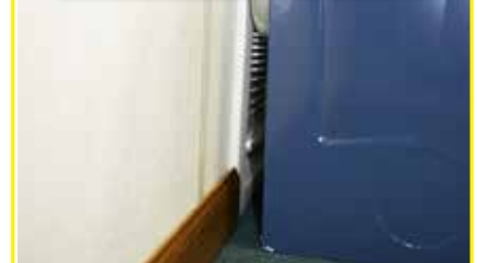
③ Dryer is close without crushing duct
